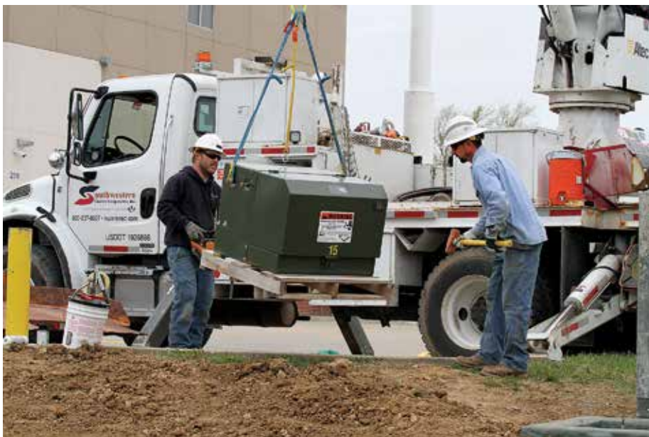
Tyler Isaak (left), construction foreman, and Jimmy Revisky, apprentice lineman, position a transformer for a ChargePoint Level 3 charging station. In an hour, the station can provide enough charge for an EV to cover about 250 miles.
