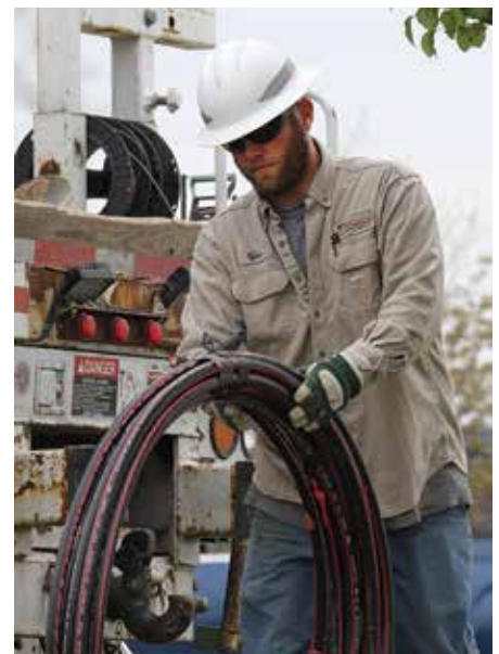
Tyler Kunz, journeyman lineman, prepares underground cable for the new charging stations.
