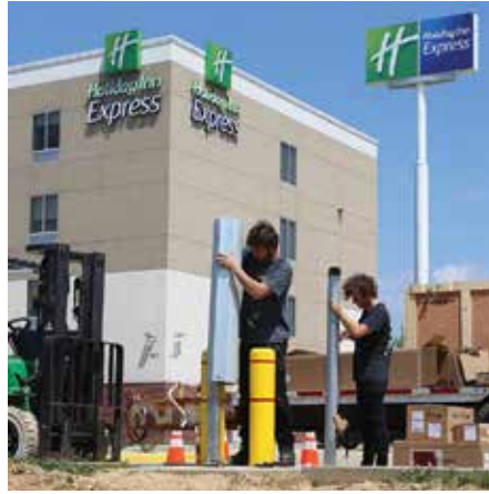
ChargePoint operates the world's largest network of independently owned EV charging stations. Above: installation day.
